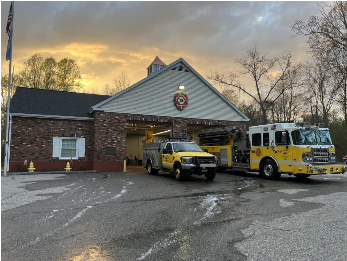
Company Two Substation – 424 Westchester Road - Westchester
